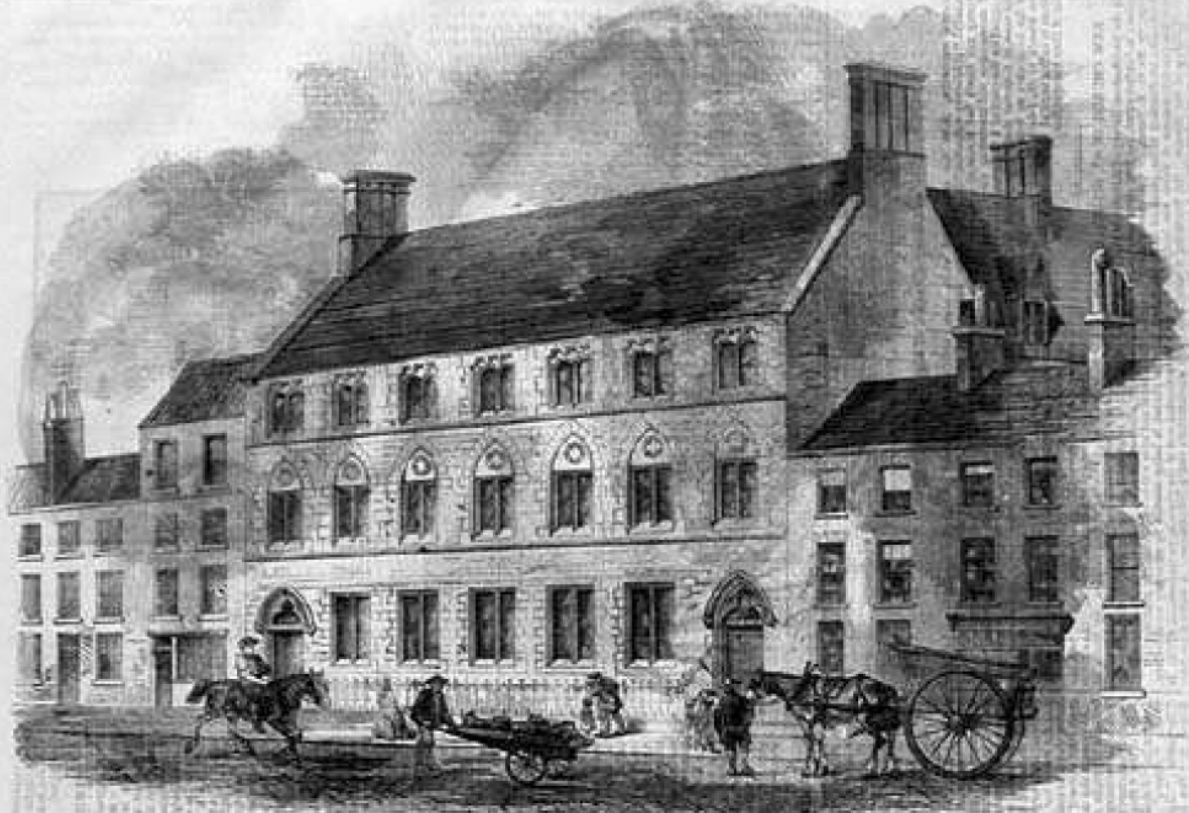
NATIONAL, INDUSTRIAL, AND SEAFAR SCHOOL OF ST. JOHN THE BAPTIST.—THIS NEW 12-ROOM SCHOOL, FRONTING SQUARE
