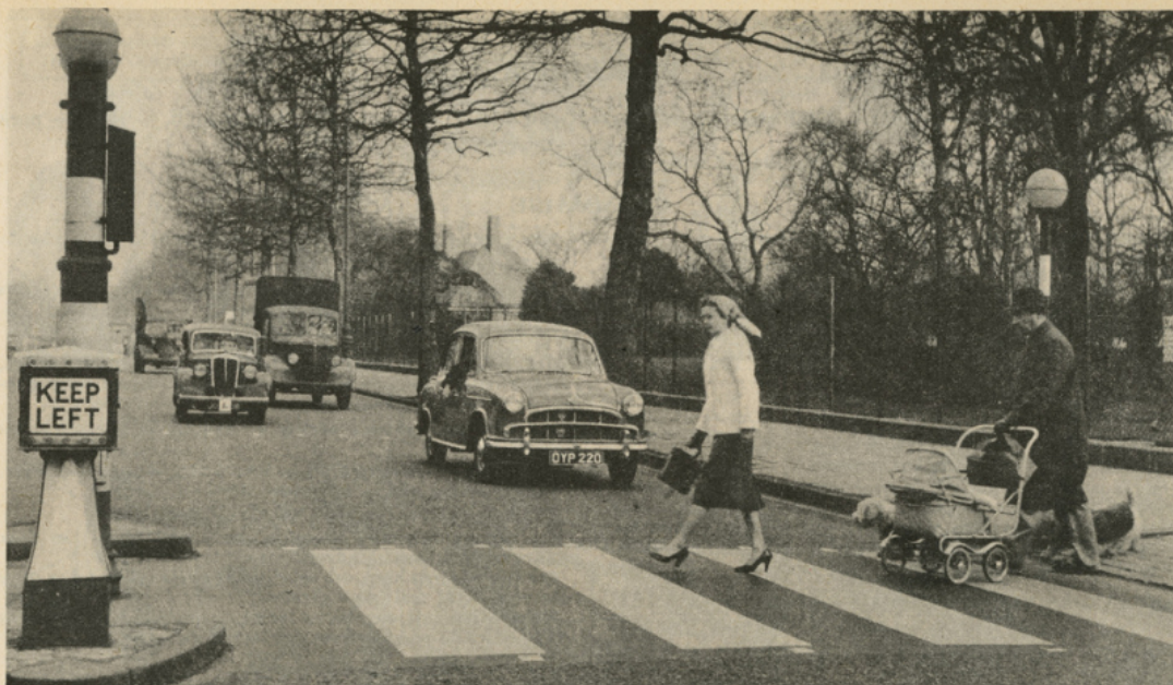
TRAFFIC ISLAND, KEEP LEFT SIGN, ZEBRA CROSSING AND BEACON
